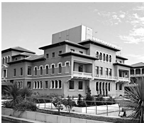
Fig. 1. Building 16, the Library is on the second floor.
